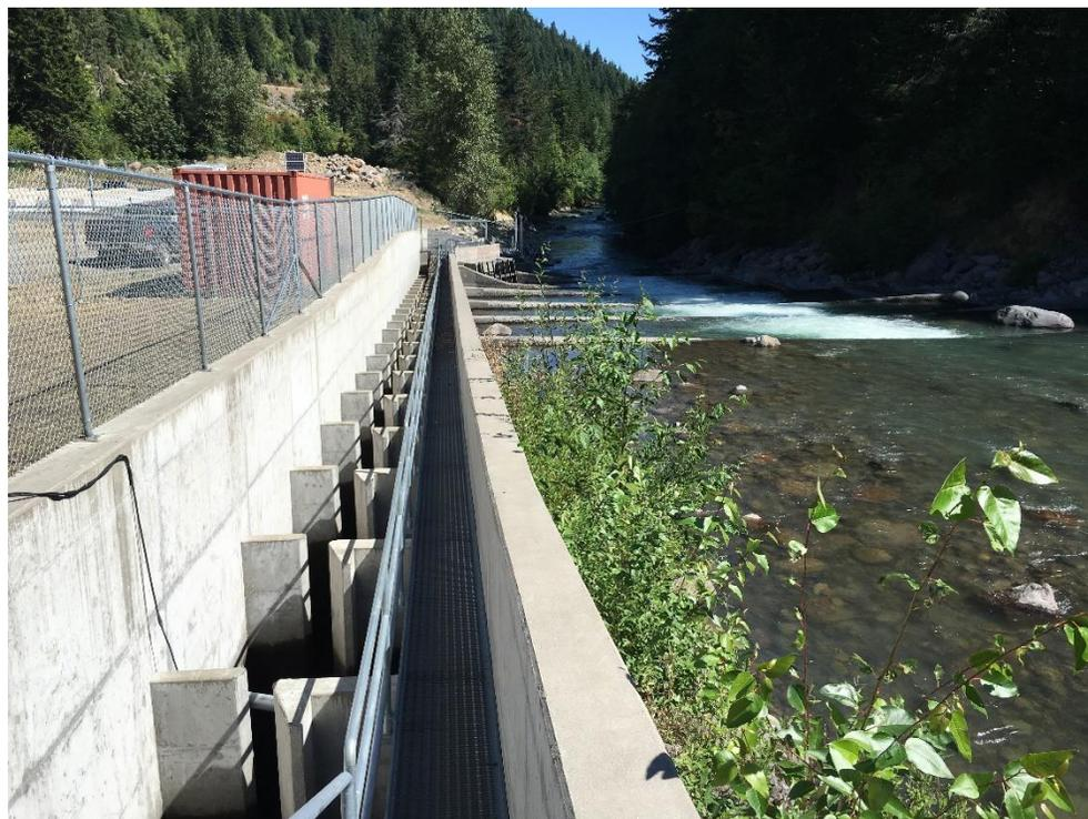
Figure 4: Fish ladder located on the Hood River in Oregon, allowing salmon passage around a small obstruction in the main channel of the river. Water flows down the channel, but its flow is slowed by the concrete barriers. Such structures can help fish navigate smaller obstacles but are often not feasible options for allowing passage around larger dams.
